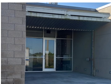
DeSoto County EOC before installing impact glass
