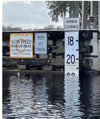
Post-storm water level under Astor Bridge
