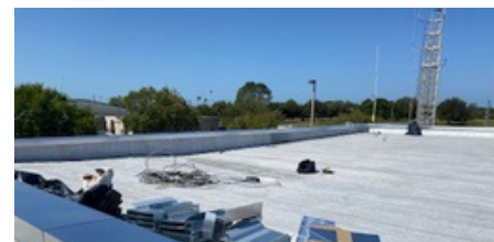
DeSoto County EOC after roof replacement
