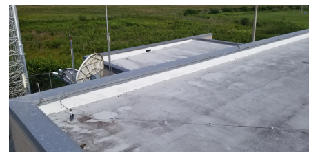
DeSoto County EOC before roof replacement
