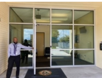
DeSoto County EOC after installing impact glass
